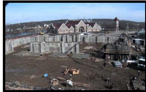
*Beams are being placed underneath the National Czech & Slovak Museum & Library building as it is being prepared to move to the new foundation being constructed in the foreground. Webcam views can be seen at [www.NCSML.org](http://www.NCSML.org).*
